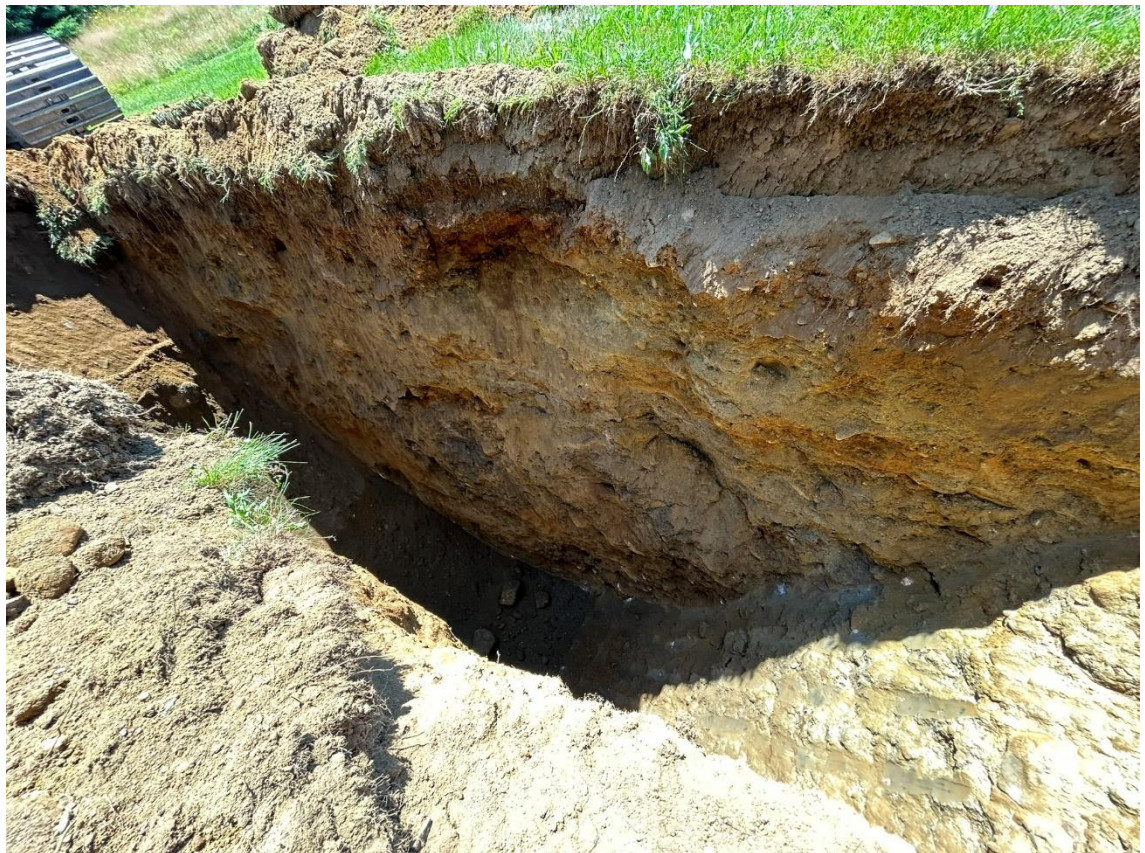
Photograph 2: Test Pit 2. July 19, 2024.
