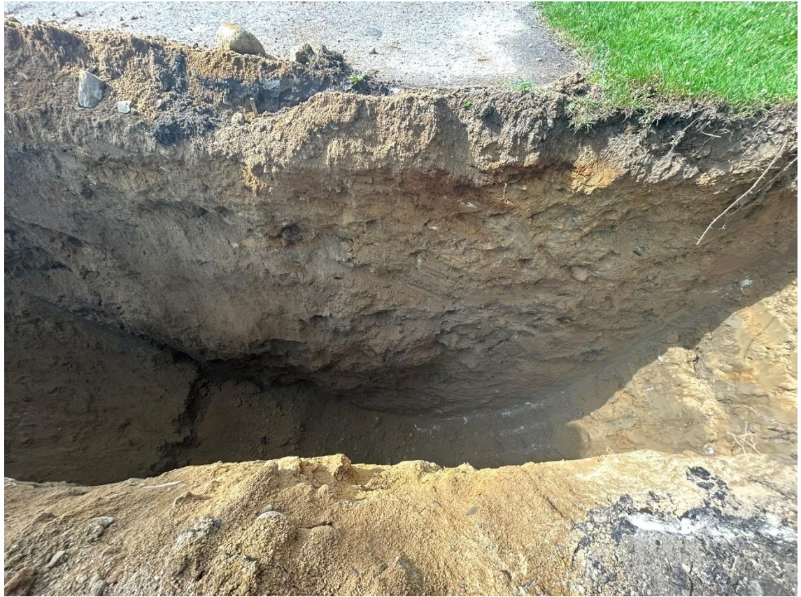
Photograph 1: Test Pit 1. July 19, 2024.
