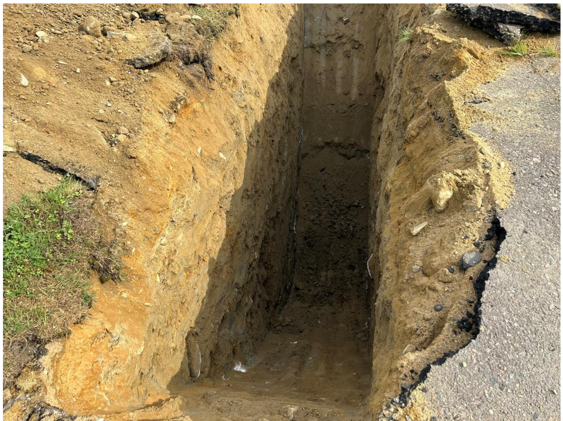
Photograph 4: Test Pit 4. July 19, 2024.
