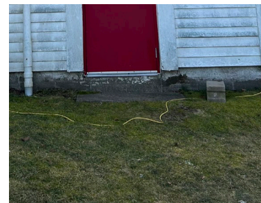
Foundation at Side Door
