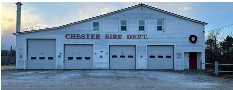
Service Apron to Bays
