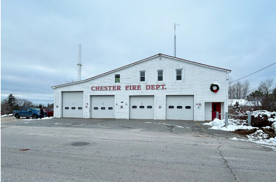
Existing Fire Station
