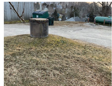
Back Gravel Pad
