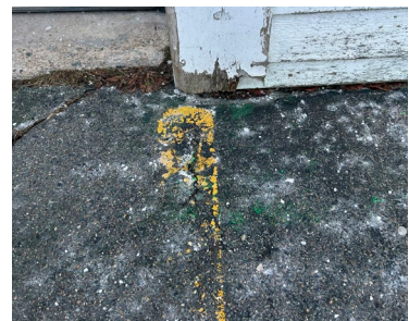
Asphalt at Building
