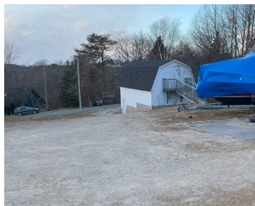
Back Gravel Pad and Shed
